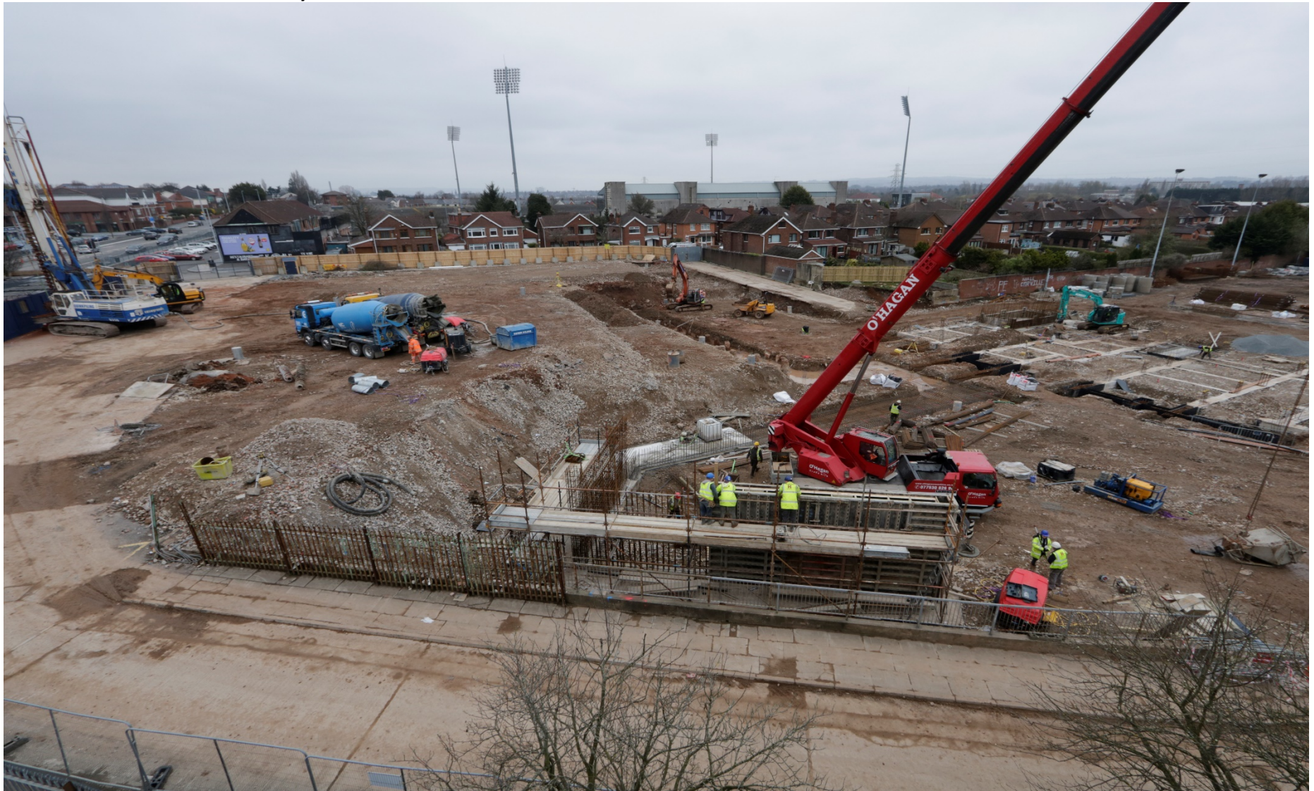
Andersonstown – Works Underway – March 2018
